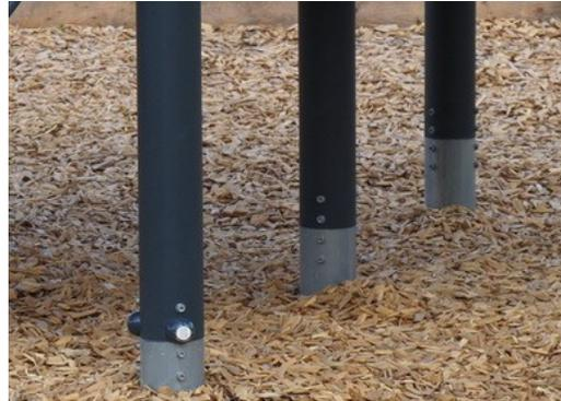
Main posts with hot dip galvanized steel footing are available in different materials: Pressure impregnated pine wood posts. Pre-galvanized inside and outside with powder coated top finish steel posts. Lead free aluminium with color anodized top finish.
