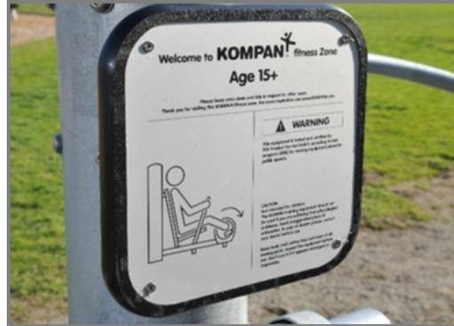
The sign consists of a 1.5mm aluminium plate with serigraphy print, sealed by a subsequent anodizing process, screwed on to a machined plate of 19mm EcoCore™.
